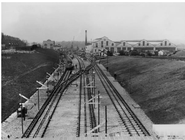
Constructing Golders Green station (c. 1904) Credit: London Transport Museum
